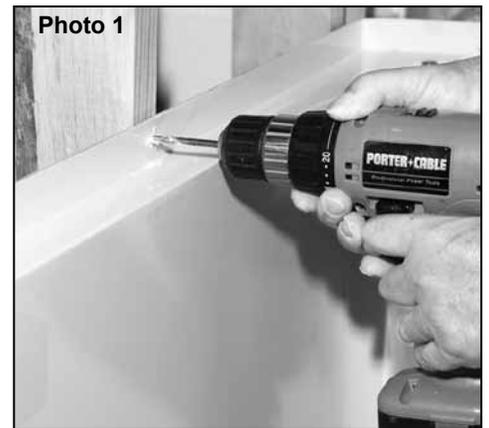
2a. With the leveling material cured and the base component securely attached to the framing, dry-fit the mid-section to confirm proper alignment, and identify any required shim adjustments necessary for the base component.
