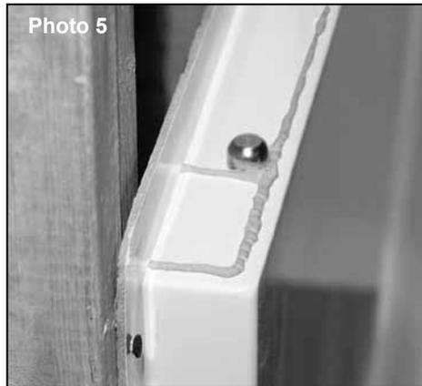
3. With the mid-section securely attached to the framing, repeat the dry-fit process with the top-section to confirm proper alignment, and identify any shim adjustments required to the mid-section. (Refer to and follow steps 2a, 2b and 2c for detailed instructions, and supporting notes to complete the assembly of the top-section.)
